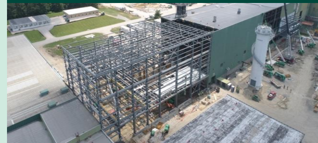
BUILDING EXTENSION - JUNE 2022
