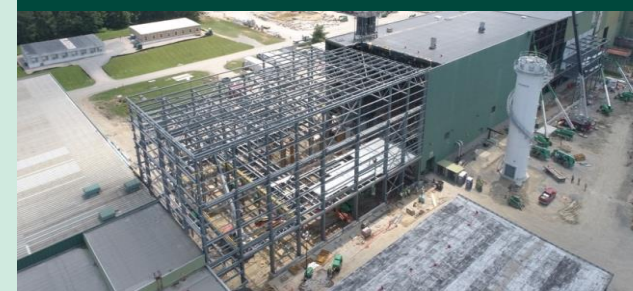
BUILDING EXTENSION - JUNE 2022
